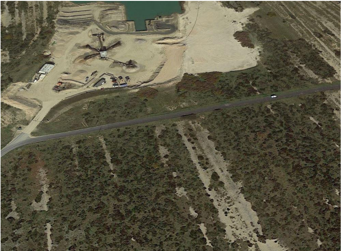
AP 2. View of Kirton Road and industrial works (looking north)
